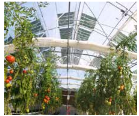
OET's OPV installations in an agricultural green house
